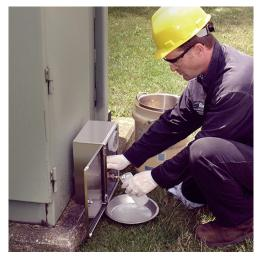
Figure 5 External Oil Sampling -Courtesy SDMyers
