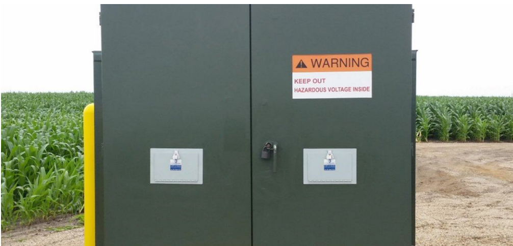
Figure 13 One large format Maintenance Inspection window is fitted on the LV side and another on the HV side of an Oil-Filled Pad Mount transformer allowing for inspection of all the internal connections
